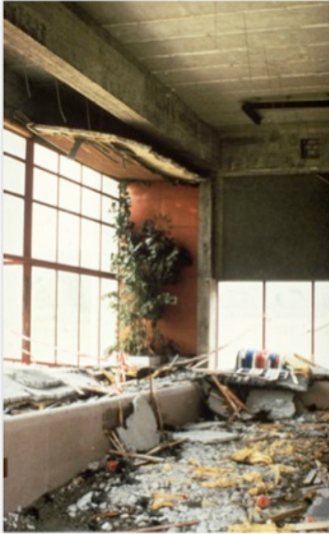
Figure 29: Collapse of suspended ceilings in swimming halls due to inappropriate stainless steel fastening elements. Failure by stress corrosion cracking. 41
